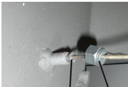
Sensor sleeve Union nut
